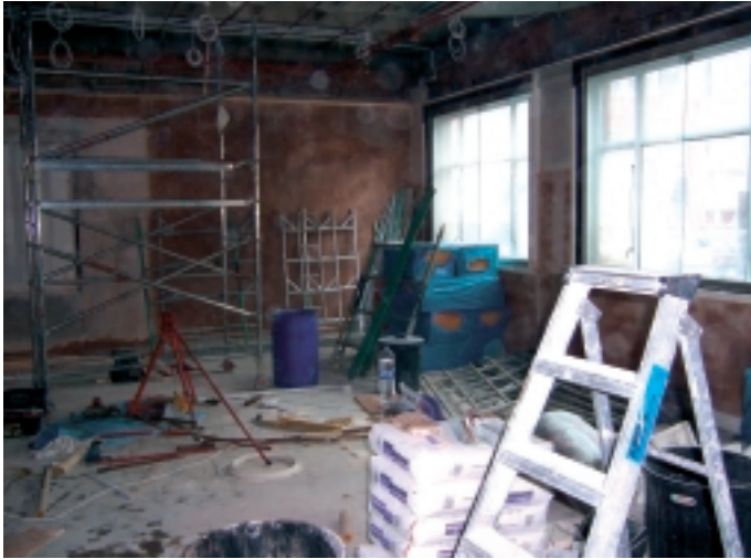
The Nuffield Lecture Theatre in the process of renovation
